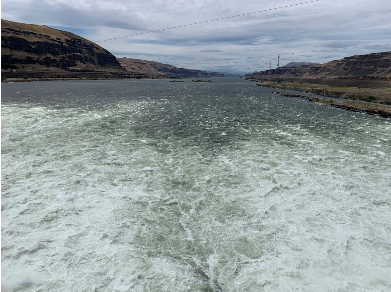
Photo taken from spill bay #11 looking downstream
